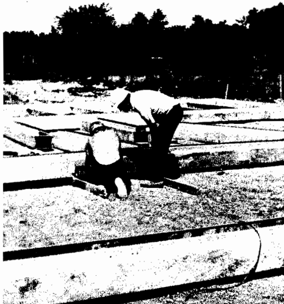
Fig. 10—Republic Steel grade beams
