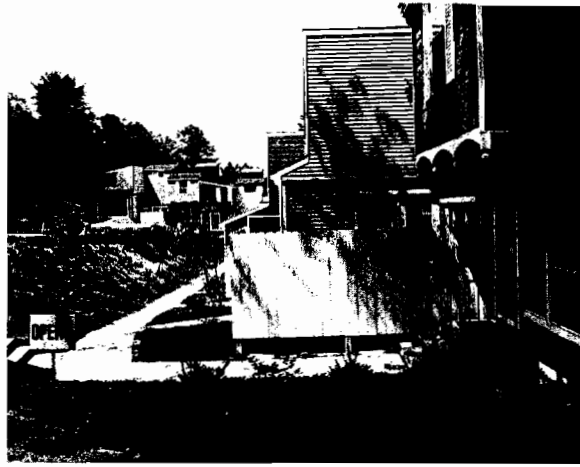
By late spring, 1972, some townhouses were ready. During the next year, the rest of the units were completed, accepted by the developer, and turned over to the marketing agency.
