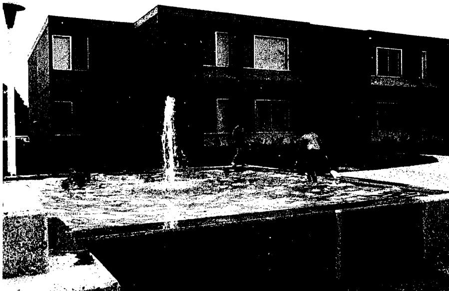
Fig. 20—General Electric units and adjacent courtyard
