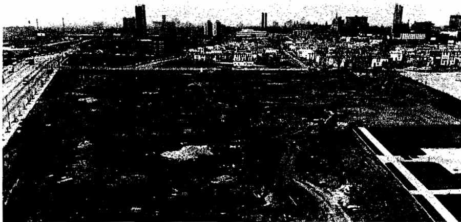
Fig. 8—The east site—view west before construction
