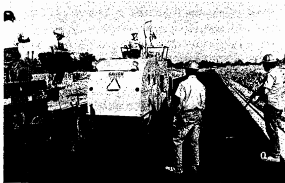
Fig. 8—Paving work preparatory to housing erection
