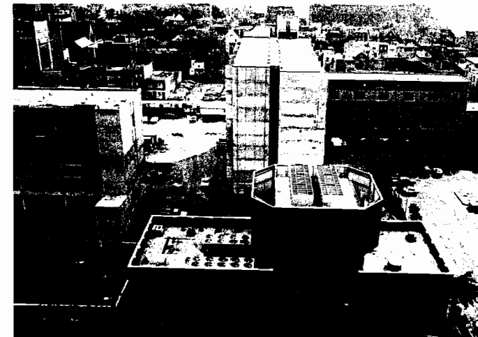
The Central Equipment Building (CEB) is at the heart of two innovative utilities systems demonstrated on the Jersey City site. The total energy system supplies electric power, hot water for heating and domestic use, and chilled water for cooling. A pneumatic trash collection system moves refuse by pipe to the CEB for compaction before pick-up.
