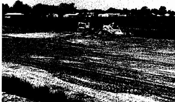
When site preparation started in the spring of 1971, an important job was the ambitious ground sculpturing, planned to give visual interest to the existing flat terrain.
