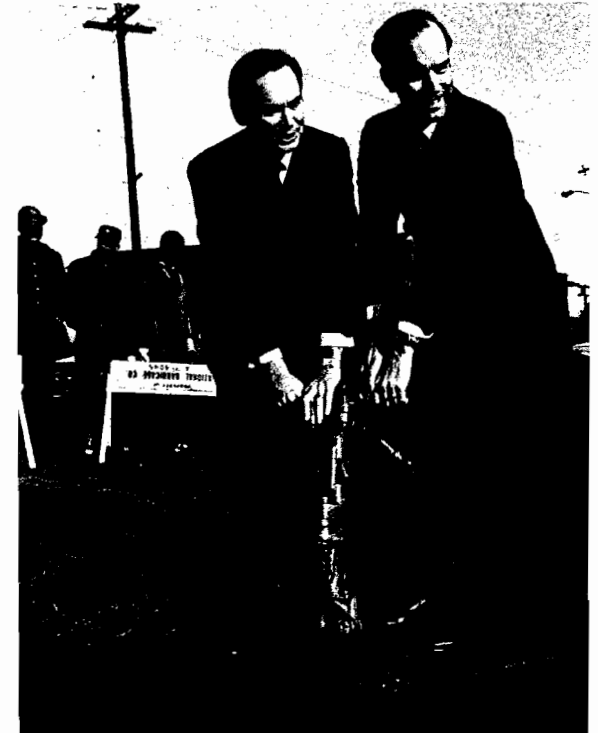
Fig. 9—Finger and Evans break ground at Seattle
