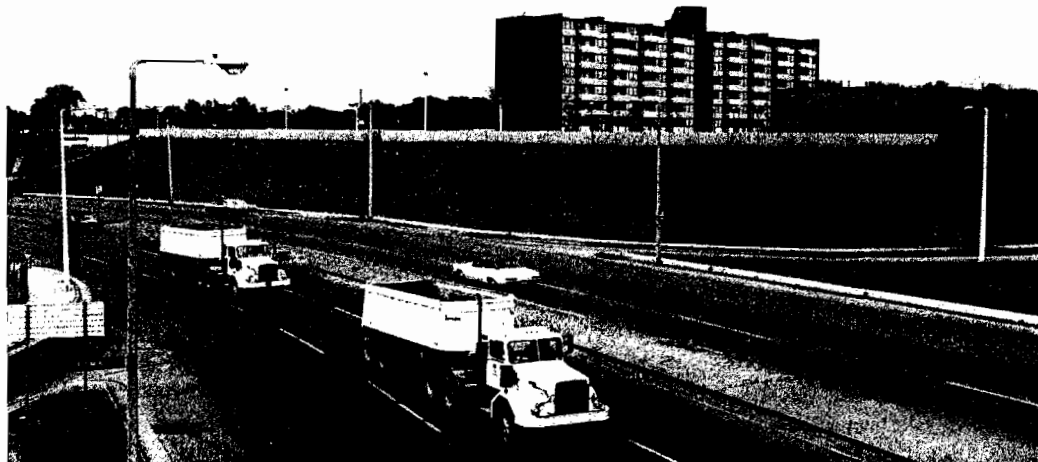
Traffic noise is controlled by an acoustical berm along Danny Thomas Boulevard. The berm is a grassy, earthen barrier with a low concrete wall along its crest. Together, these absorb and deflect sound, reducing the noise level on the site.
