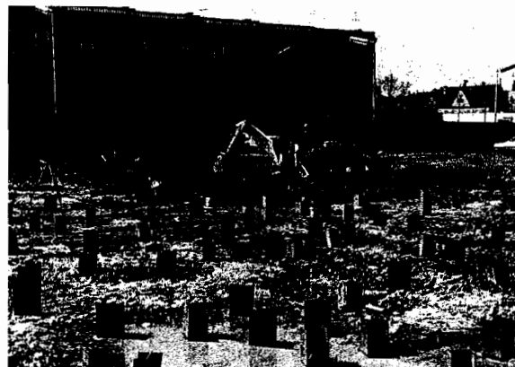
Fig. 18—Piling for CAMCI high rise
