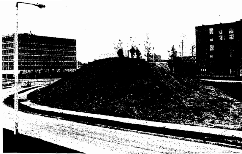
Fig. 23—Berm at southwest corner of site
