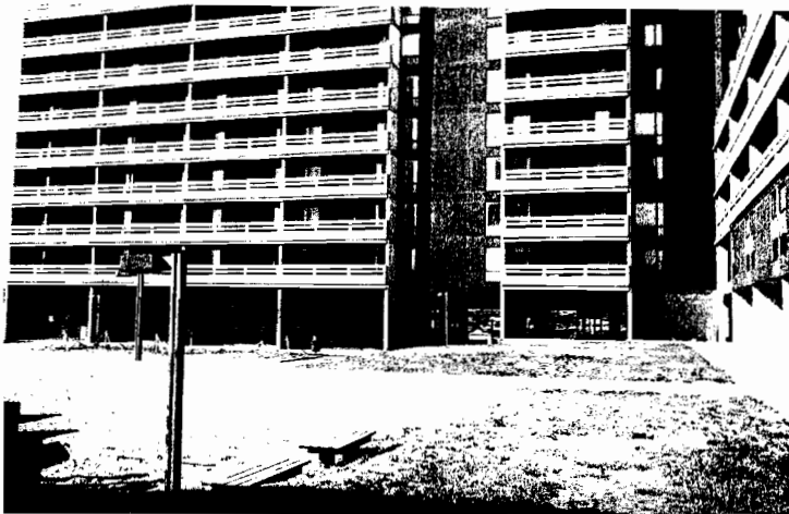
Fig. 19—Completed Descon high rise
