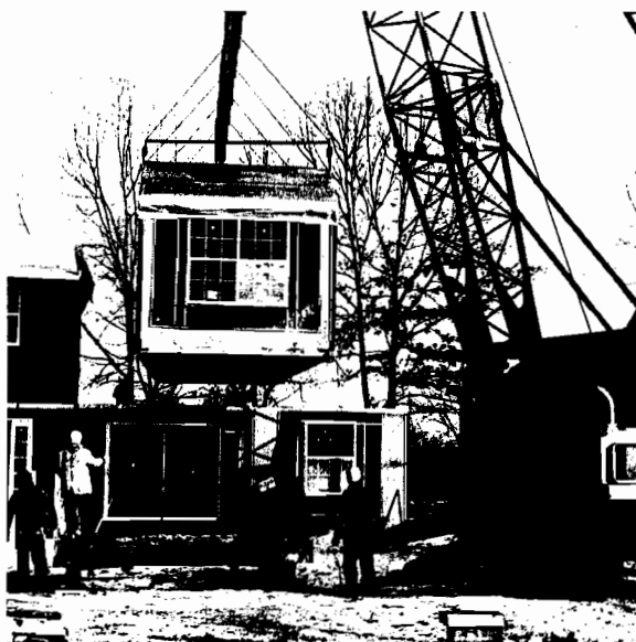
Housing construction at Indianapolis began in August 1971 and continued through the difficult winter weather. Six of the eight systems used volumetric modules, which lend themselves to rapid erection. Finishing operations extended completion of all 295 units until mid-1973.
