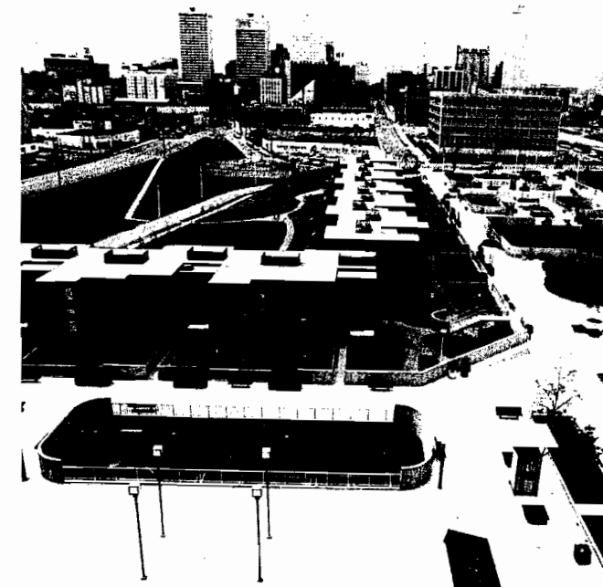
East of the acoustical berm a spine, or pedestrian platform, provides open space for recreation and community activities while covering a parking area. It also serves as a pedestrian pathway between the medical center and downtown.
