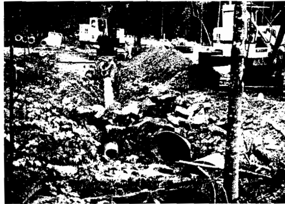
Fig. 12—Creek drained under loop road near NE 148th St.
