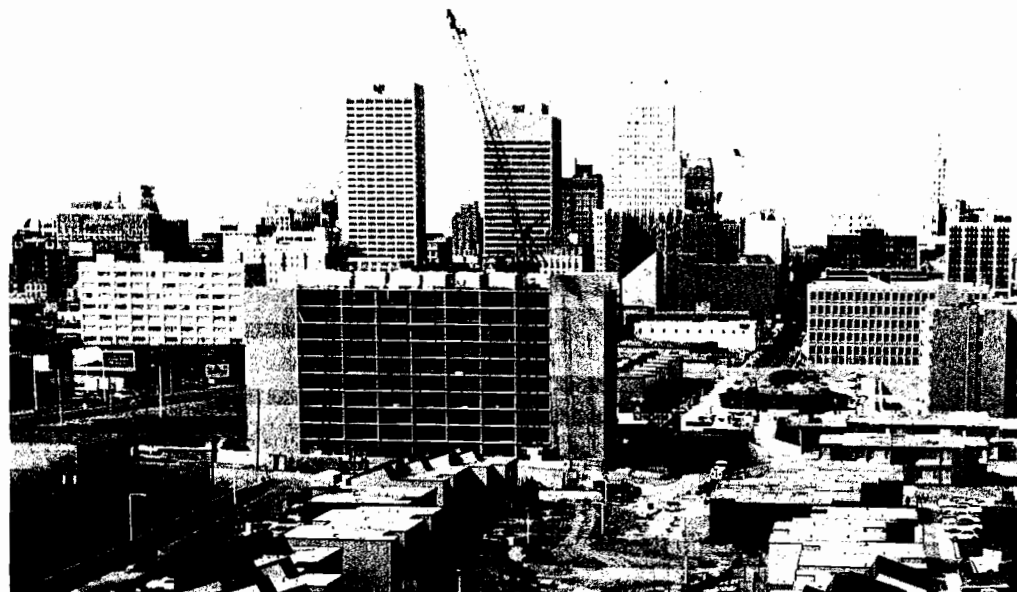
Fig. 16—Topping out FCE-Dillon high rise, March 1973
