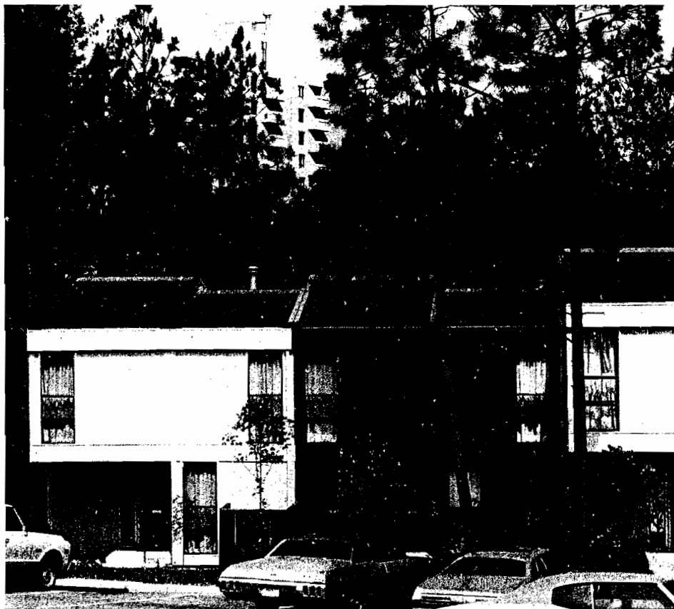
Fig. 21—Boise units across lake from high rise
