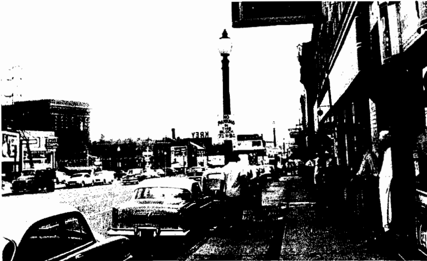
Fig. 3—Mill Creek before renewal
