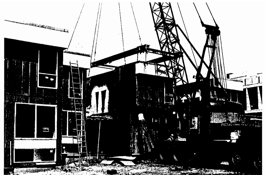
Fig. 14—Erecting a Boise Cascade townhouse
