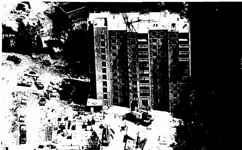
Fig. 8—BSI tower one day before topping out
