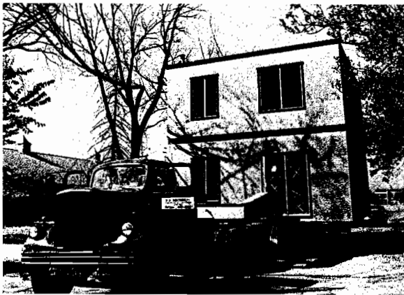
Fig. 12—Transporting CTC unit from factory
