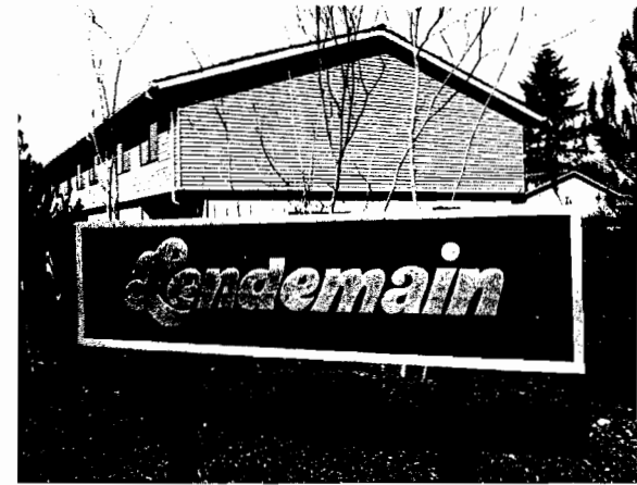
The first Lendemain homes went on the market in July 1972. Initial sales were slow, partly because of a limited variety of completed units. By the end of 1973, 75 percent of the units had been sold on the open market in a price range compatible with values in the surrounding neighborhood.
