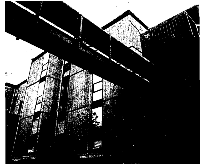
Fig. 22—Boise Cascade units with connection to spine
