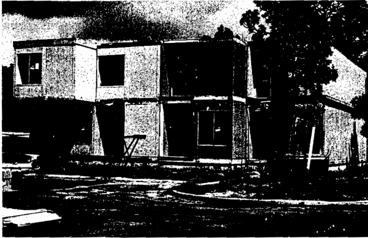
Fig. 10—Erected MSC townhouses ready for finish work
