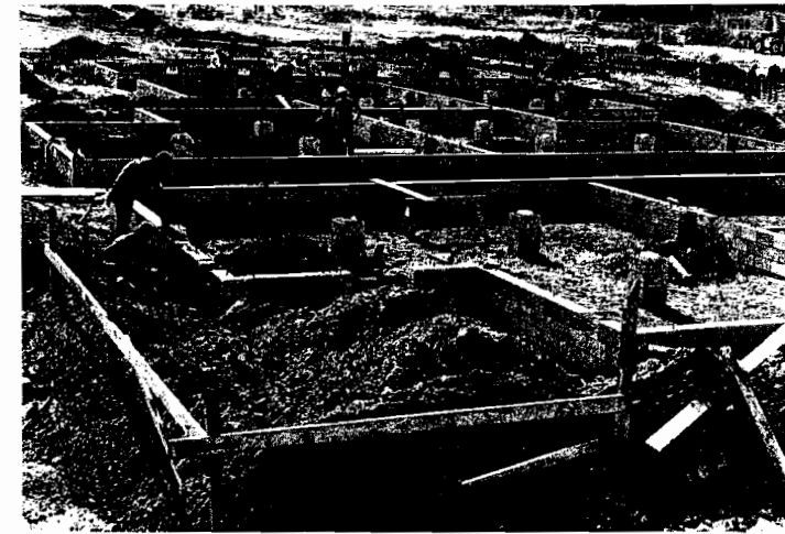
Fig. 12—Boise Cascade townhouse foundations
