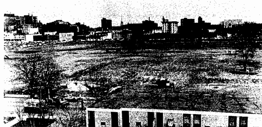
Fig. 9—The west site—view north before construction
