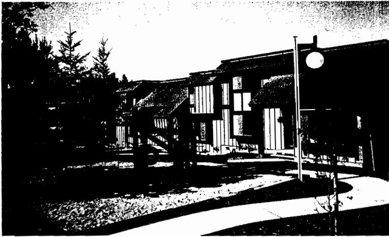
Fig. 22—Finished Levitt units and tot lot
