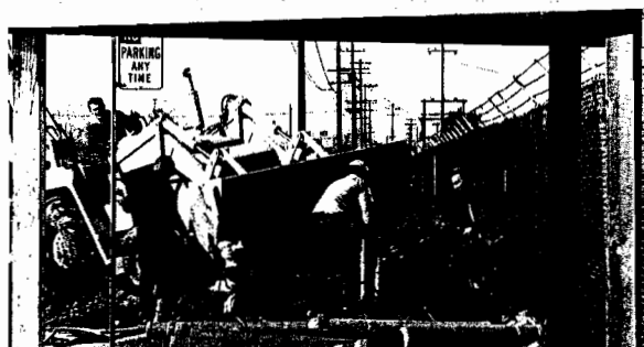
Fig. 6—Sewer installation along Broadway
