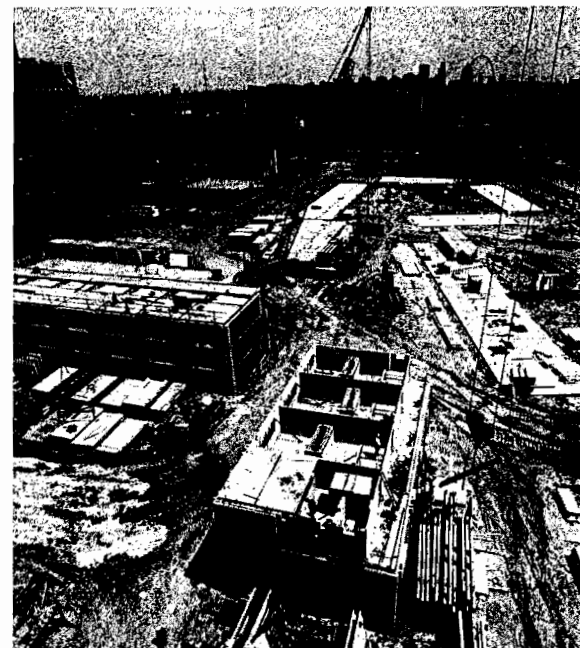
Site preparation started in November 1970 and, strengthened by the broad participation of minority and non-minority businesses, housing construction was well under way by the end of 1971.
