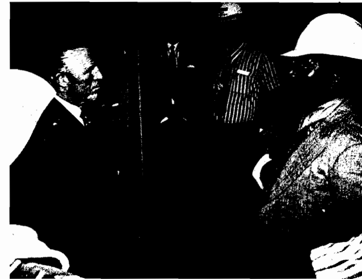
Fig. 5—Former HUD Secretary Romney meets subcontractors
