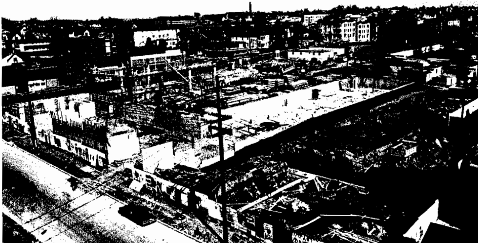
Fig. 10—Initial on-site construction
