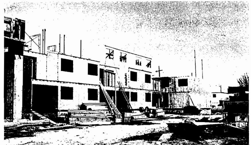
Framing for the housing units is an adaptation of the Rusco system. Factory-cut to size and identified as to final location, the steel channels were assembled using sheet-metal screws and a limited amount of welding. Wall surfaces are conventional, with gypsum board inside and cedar siding over plywood outside.
