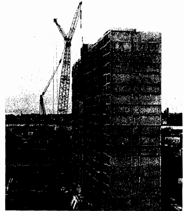
Fig. 20—Shelley A topping out, April 1973
